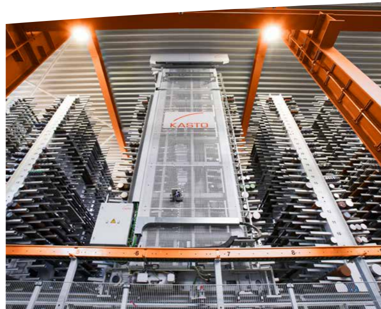
Operating gantry crane in portal design with maintenance walkway.
